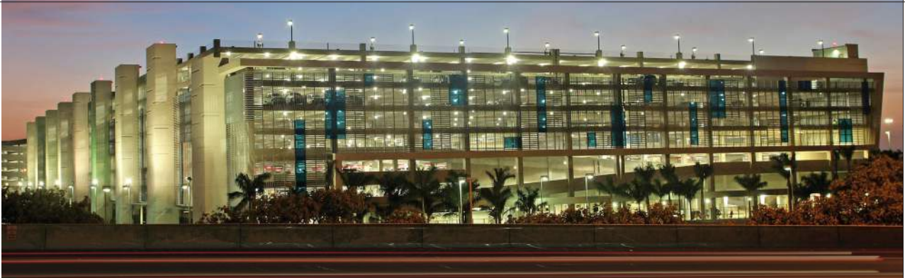
The Cypress parking garage at Fort Lauderdale-Hollywood International Airport was the first facility to earn Parksmart's Pioneer certification. An advanced, efficient HVAC system, valet EV charging, and tire-inflation stations are a few features of the parking structure.
